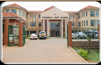
Commercial Court Building Temple of Justice
