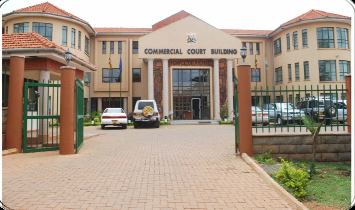
Commercial Court Building Temple of Justice
